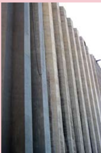
Work in progress on the silo repair project in Randfontein.
