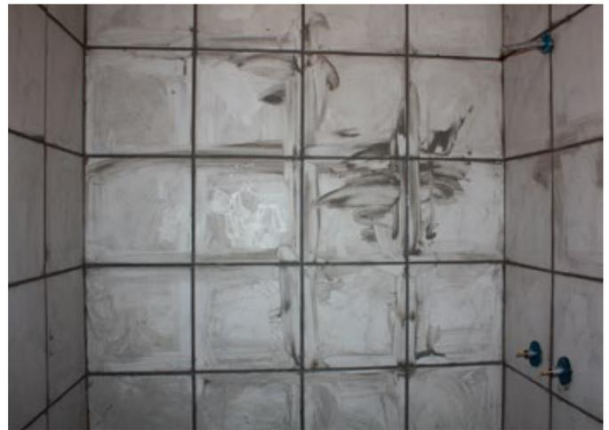
Coverage: (3kgs/m2 total system i.e. 1kg/m2 per coat – 3 coats required)
