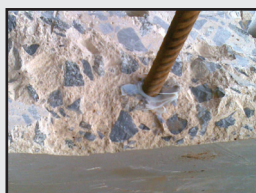
FOR GROUTING VERTICALLY DOWN
