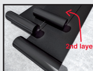
STEP 2 DOUBLE LAYER COVERING
