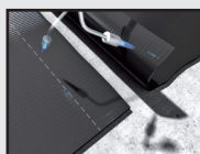
STEP 1 SHEETS GET TORCHED ONTO SUBSTRATES
