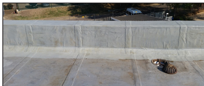
One coat of abe.® proof liquid membrane applied to parapet.
