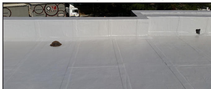
One coat of abe.® proof liquid membrane UV topcote applied to substrate.
