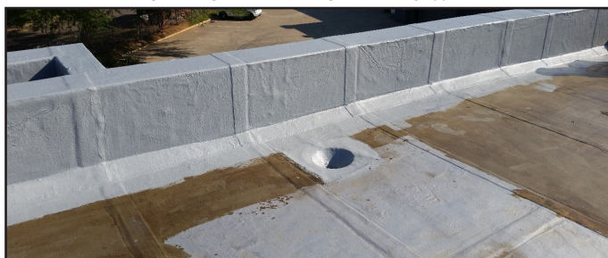
Second coat of abe.® proof liquid membrane primer applied to parapet.
