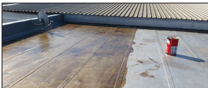
One coat of abe.® proof liquid membrane primer being applied to the substrate.
