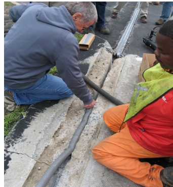
Placing the backing cord
