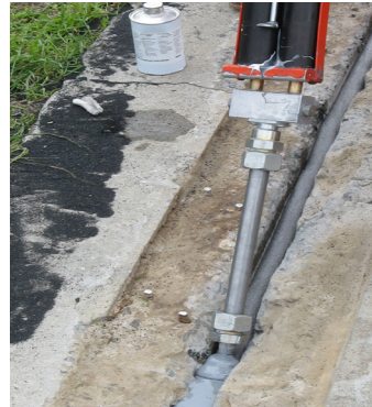
Applying the sealant
