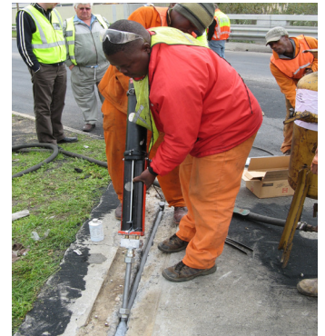
Applying the sealant
