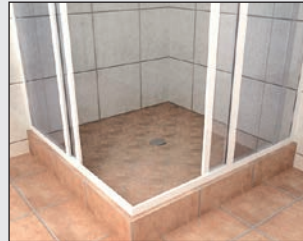
Waterproof shower before tiling
