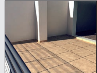
Waterproof balconies and terraces
