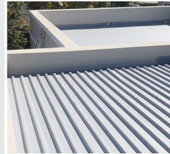
IBR & Concrete Roofs
