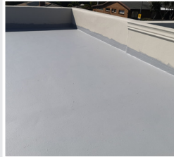
Parapet Walls & Flashings
