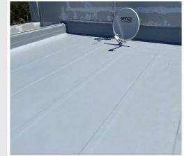
Over existing Torch-on
