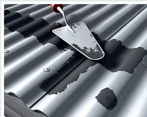
Roof laps and roof screws
