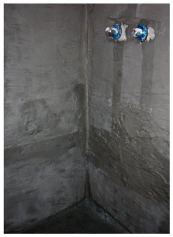
Coverage: (3kgs/m<sup>2</sup> total system i.e. 1kg/m<sup>2</sup> per coat – 3 coats required)
