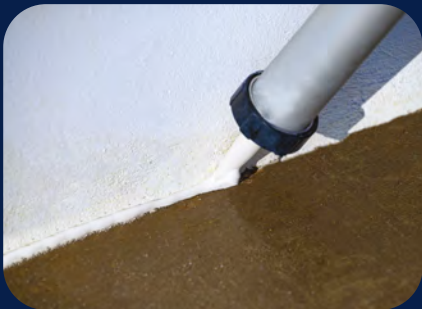
STEP 3 Fixing cracks and joints
