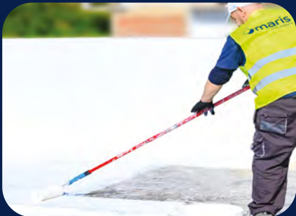
STEP 6 Reinforcement and 1st layer of waterproofing membrane
