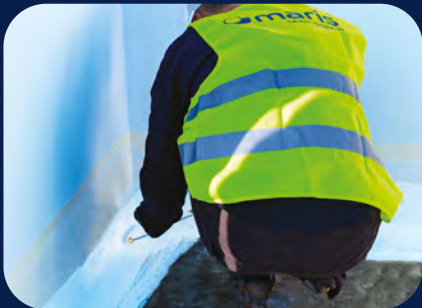
STEP 5 Wall-floor connection
