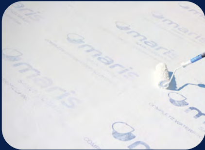
STEP 7 2nd layer of waterproofing membrane
